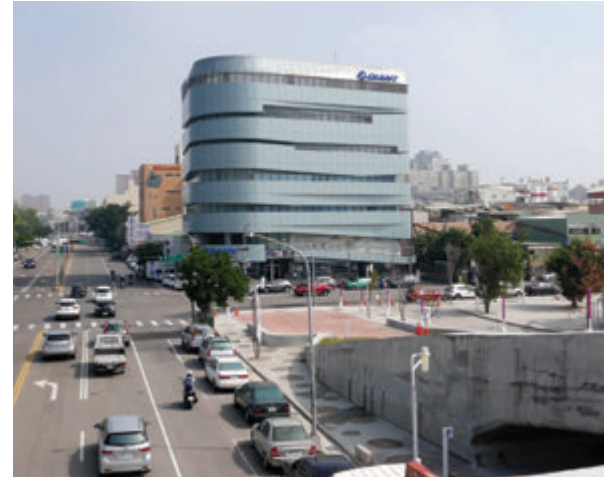
Giant's giant office building in Taichung houses its largest retail flagship store in Taiwan.
